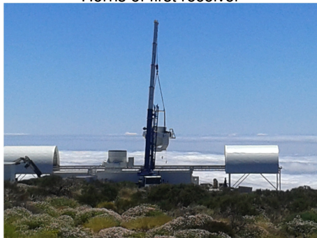
Installation of second telescope
