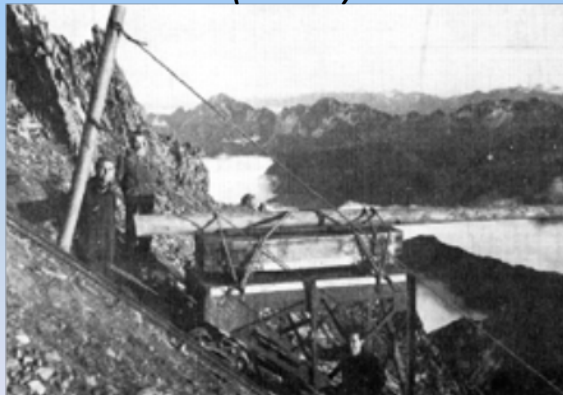
Transport of the Manchester electromagnet at Pic du Midi (1950), to be employed with the cloud chamber of Blackett e Occhialini. To install the electromagnet (only the base weight was 4 tons!), a slope 220 m , 42°, was manufactured .
